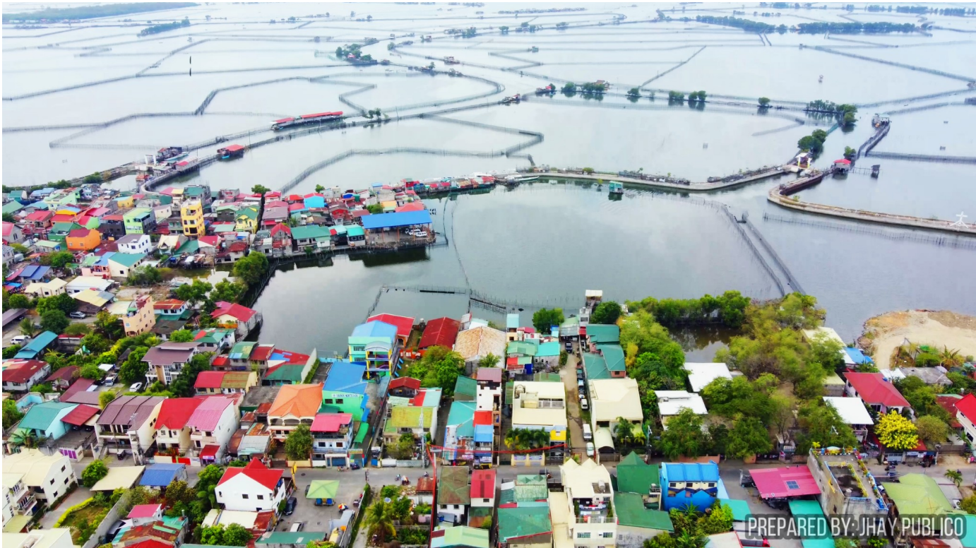
Aerial view supplied by Jhay Publico showing the property setting and surrounding community.
